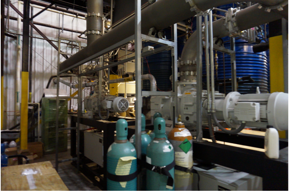
Figure 3.5: HPEPL VTF-1 Twin dual-stage mechanical pumping systems.
