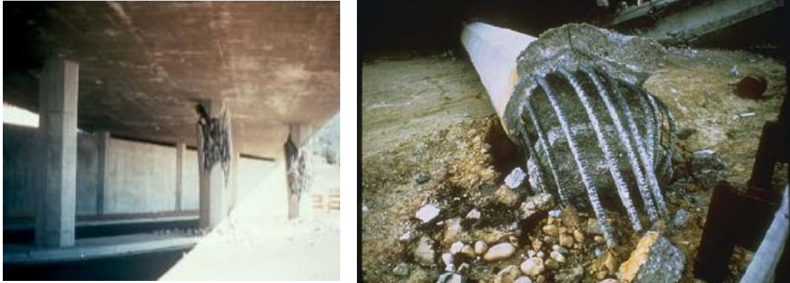
(a) (b) Figure 3. Bridge column with (a) shear failure and (b) pull-out failure in 1971 San Fernando earthquake (Veletzos et al., 2006)
