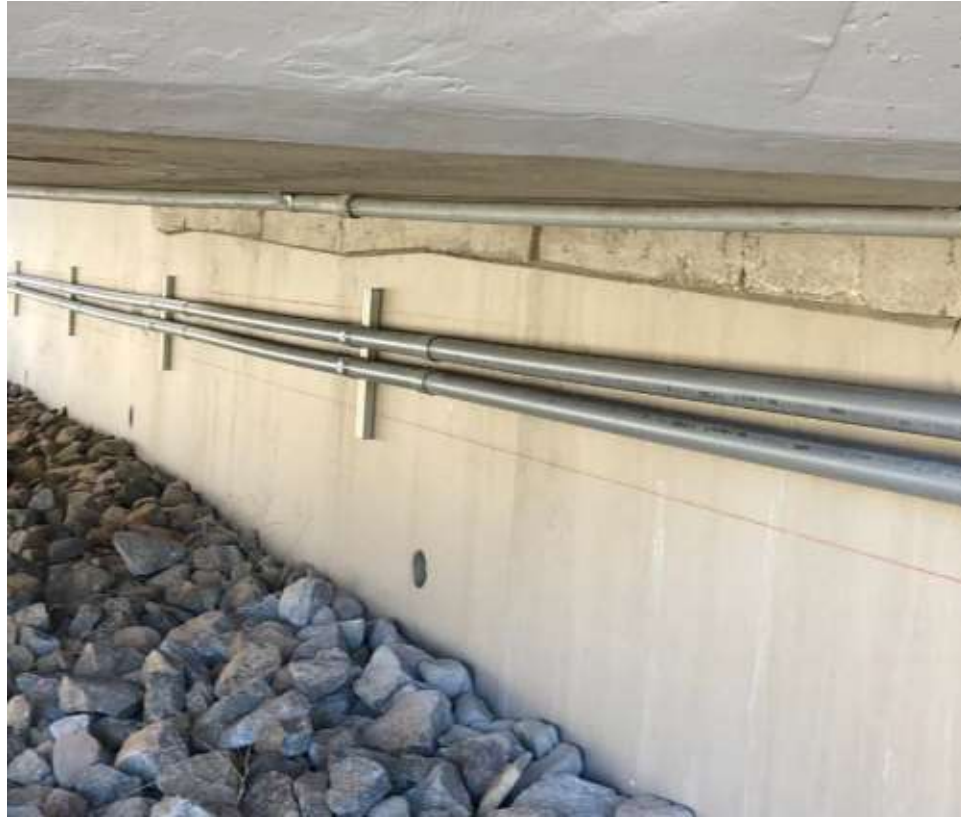
Figure 4.7: PVC conduits along the face of Abutment 1
