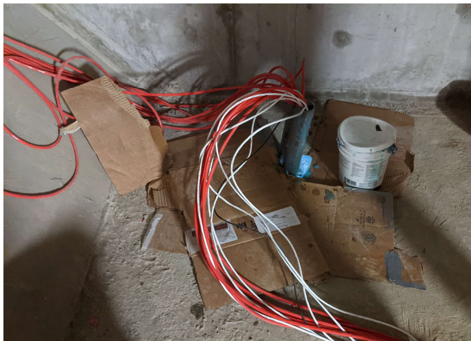
Figure 4.8: PVC conduit extruding through the bottom slab near Abutment 1
