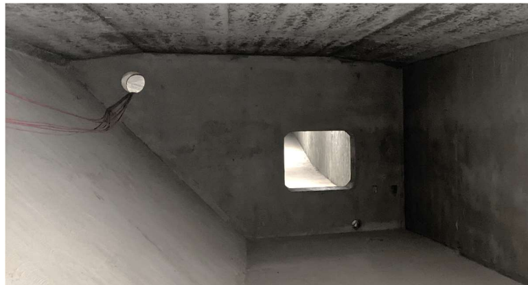
Figure 3.5: North fillet diaphragm at Span 3 of northbound structure
