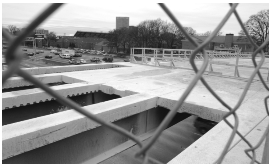
Construction crews have begun removing sections of concrete located between support beams on the southern half of the Fifth Street bridge.
