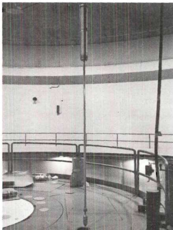
Figure 22. Dummy Fuel Element for Positioning the Detector Used in Core Position V-11
