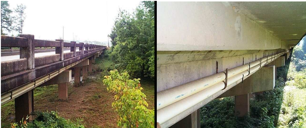
Figure 4.3 Straight T-Beam Bridge (ID: 129-0045, Gordon County)
