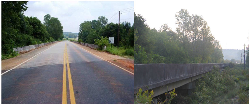
Figure 4.4 Skew T-Beam Bridge (ID: 015-0108, Bartow County)
