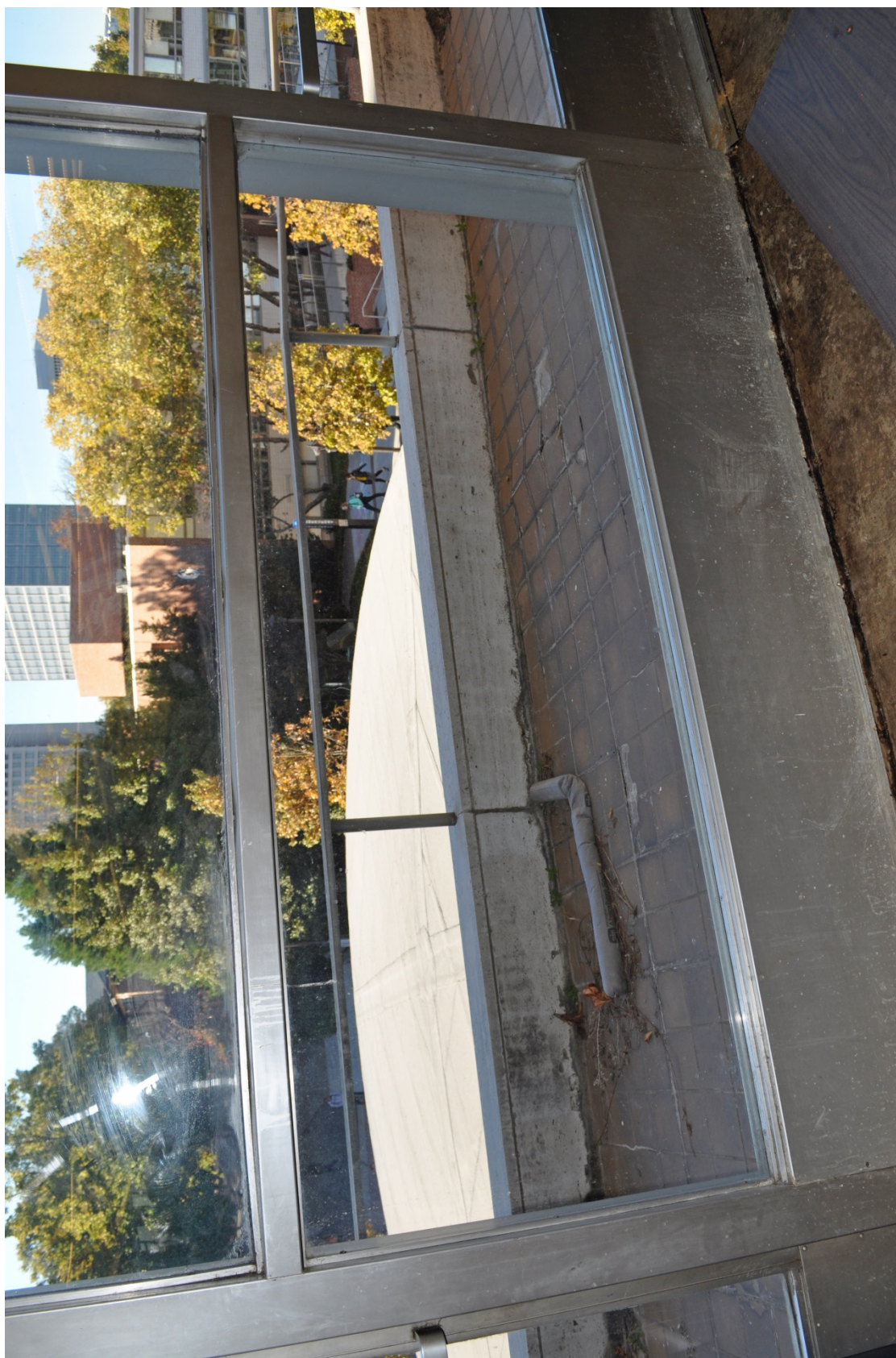
Figure 5-146: Detail of deteriorated window and door frames to balcony at third floor.
