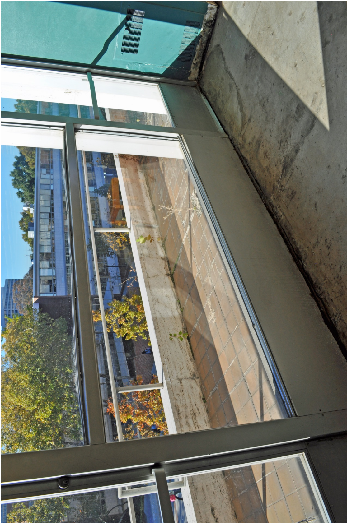
Figure 5-147: Detail of deteriorated window and door frames to balcony at third floor; note also deteriorated balcony floor.
