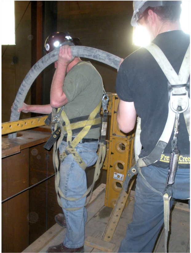
(b) Filling of the steel tubes with SCC
