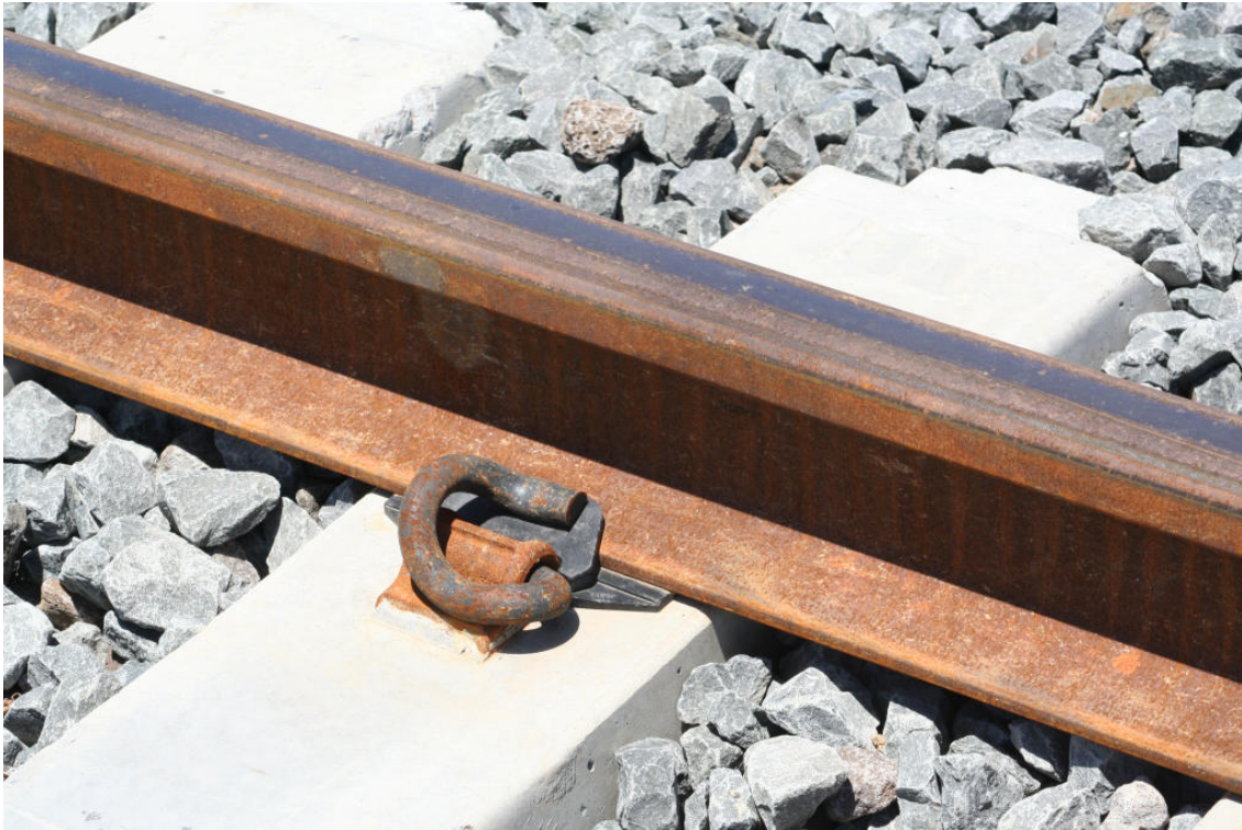
Figure 6.5: The Pandrol Fastener 350
