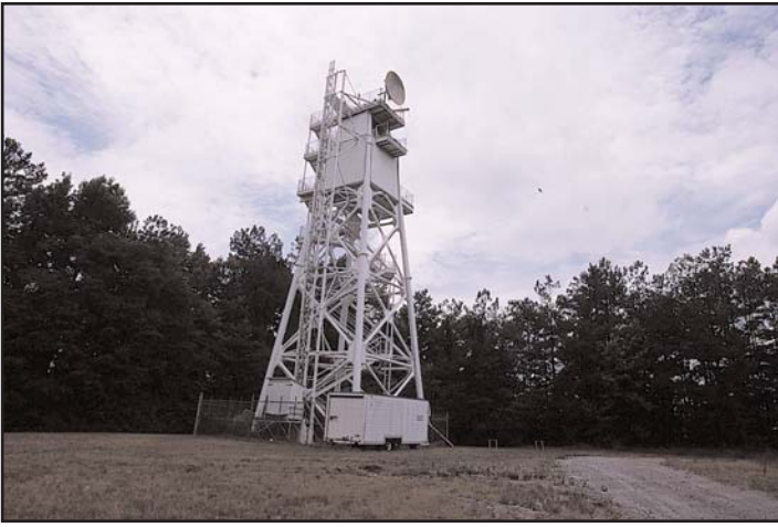
GTRI's high-precision, far-field antenna test range includes receive and source (pictured) signal towers 1,300 feet apart.
