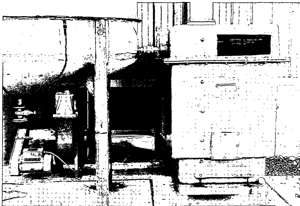
Figure 2.7 Carbon Adsorber and Fan for the Gas Clean-up System.
