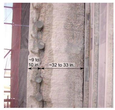
Figure 2.5: Photograph of delamination after removal of concrete for SGR opening (Performance Improvement International, 2010)
