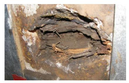
Figure 2.11: Embedded wood found in containment concrete at Beaver Valley Unit 1 after removal of corroded liner (Dunn et al., 2011).
