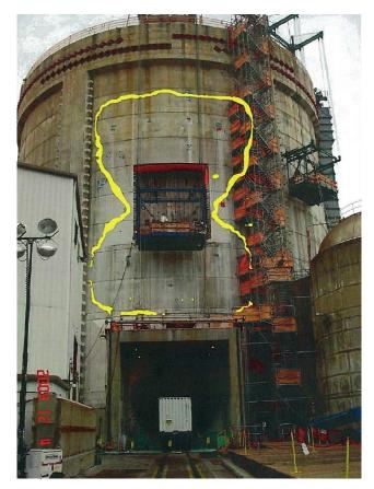
Figure 2.6: Photograph of bay 34 with overlay indicating the extent of the delamination (Performance Improvement International, 2010)
