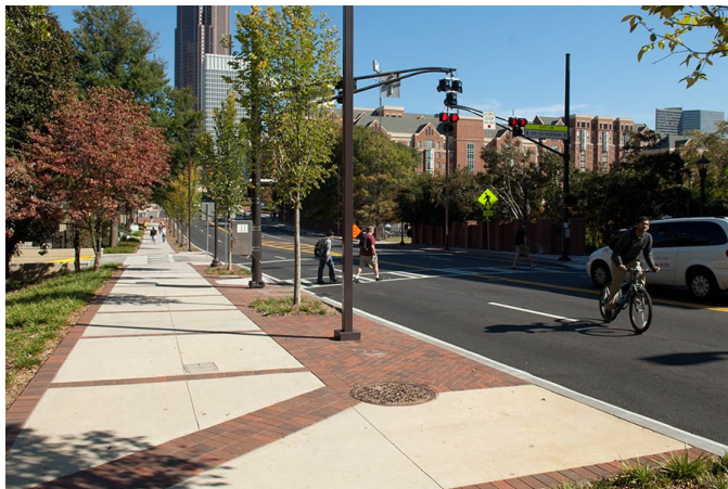
Figure 16: Good Sidewalk due to tree buffer, ample width, good pavement quality
