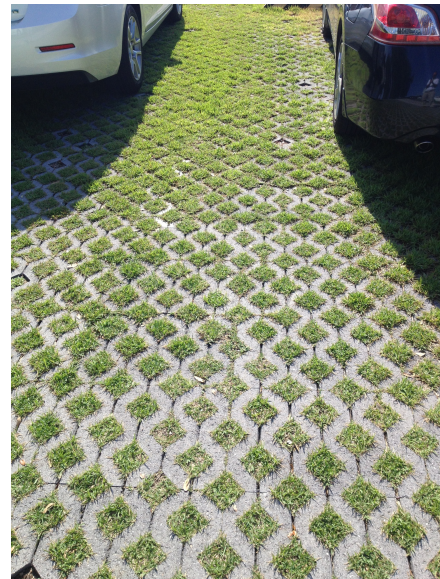
Figure 20: Pervious Pavers in parking lot VA Hospital, Orlando, FL
