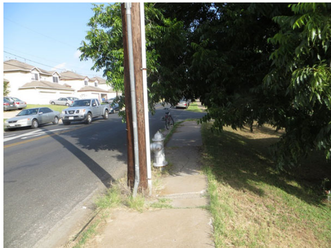
Figure 15: Poor Sidewalk due to obstructions, narrow width, broken pavement
