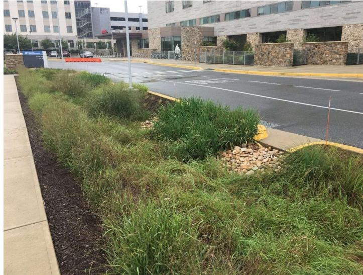
Figure 8 – Bioretention placement between curb and sidewalk (Ecological Landscape Alliance, 2019)
