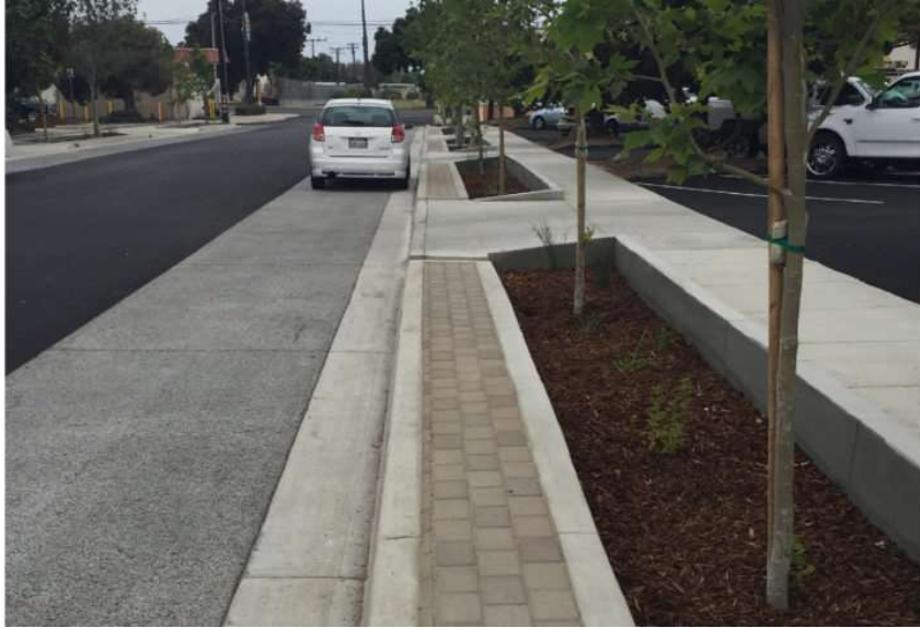
Figure 14 – Interlocking permeable pavers in the parking lane (National Association of City Transportation Officials, 2021)
