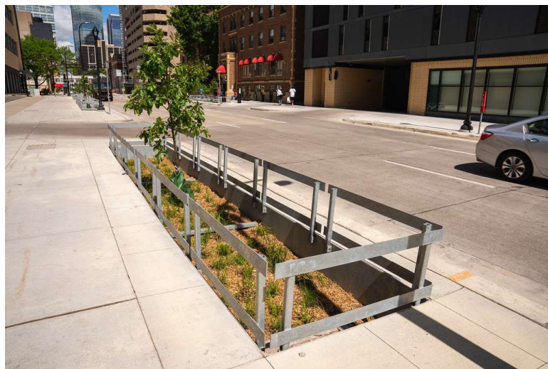
Figure 10 – A stormwater planter with a decorative railing in an urban setting (Mississippi Watershed Management Organization, 2021)
