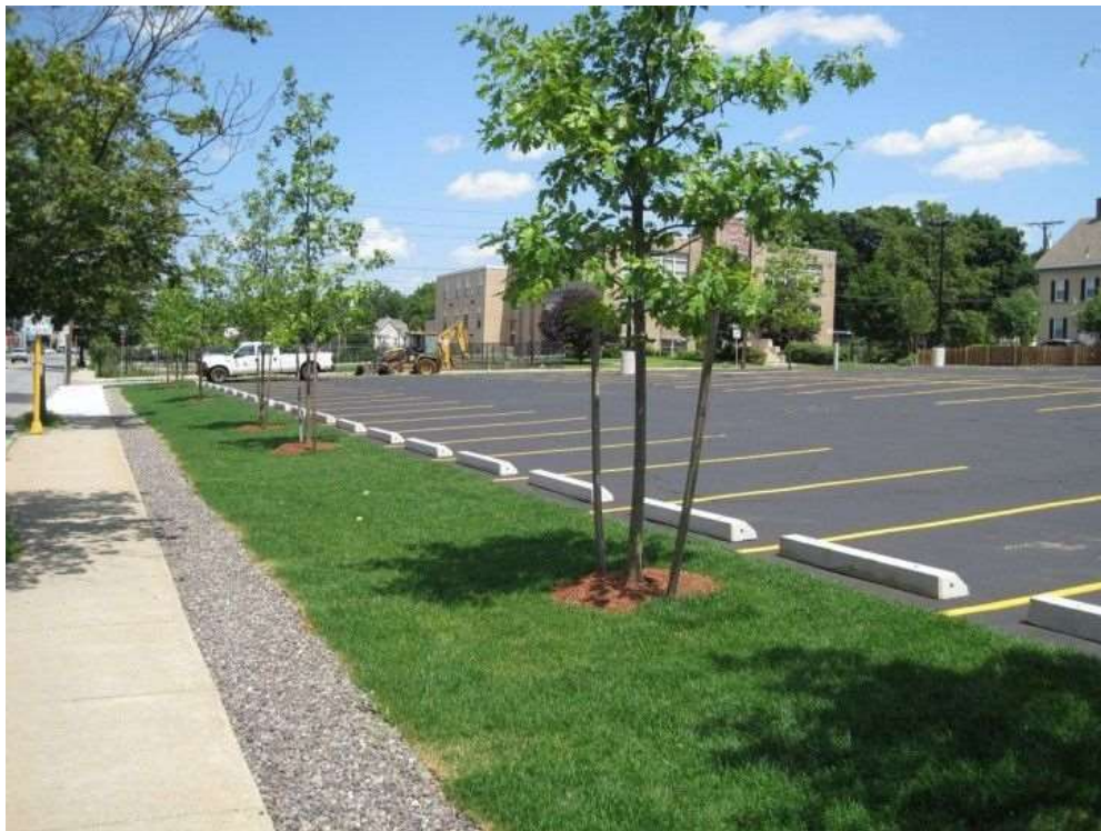
Figure 12 – Infiltration trench placement at back of sidewalk (Landscape Architecture Foundation, 2021)
