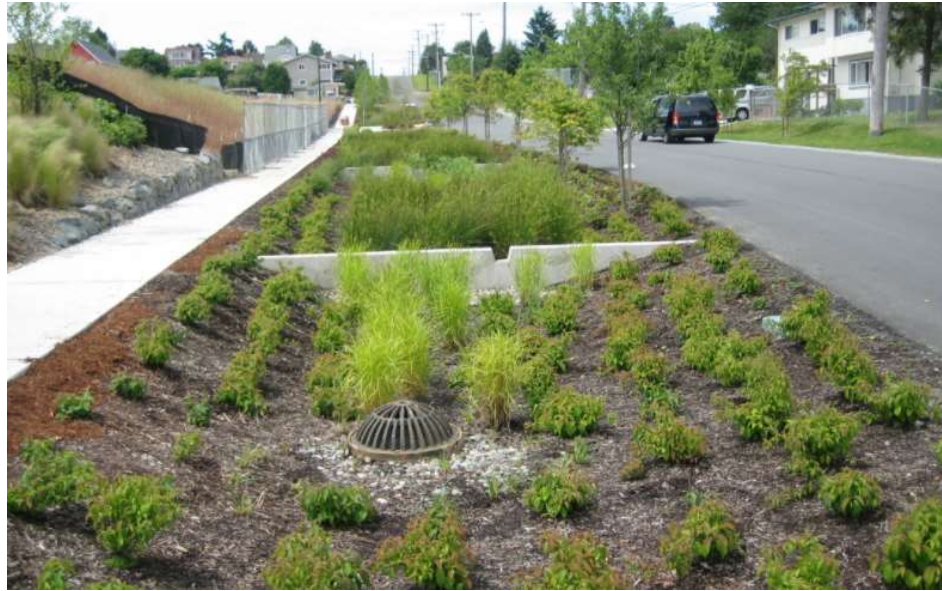
Figure 9 – Bioswale placement between roadway and sidewalk (Mark M. Holeman Inc, 2014)
